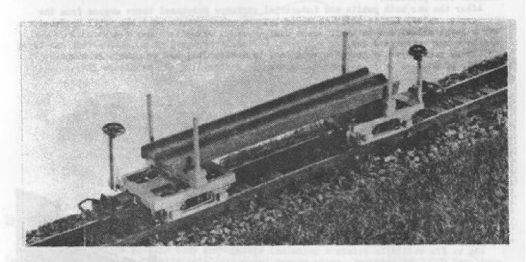
DM26 Two Hudson Single Bolster Wagons with 'H' Girder Lead
